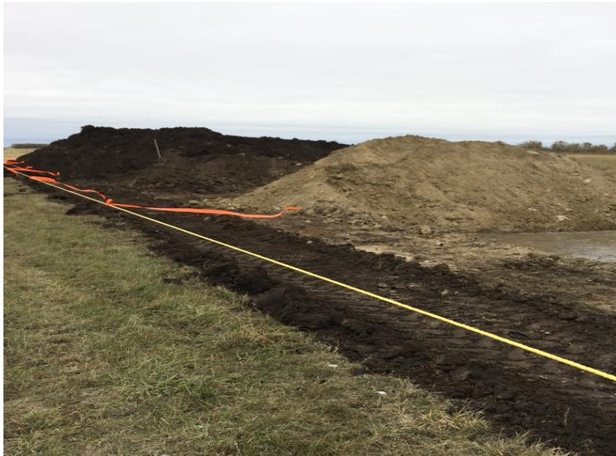
Stony Creek one of three slurry pits excavated
