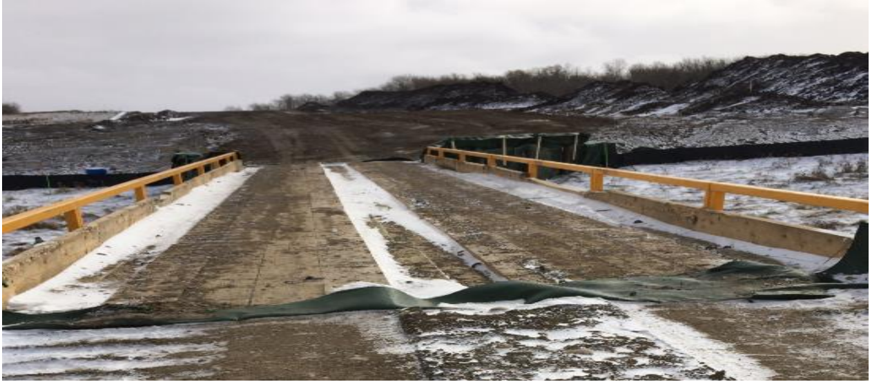
Little Pipestone Creek Bridge Installed
