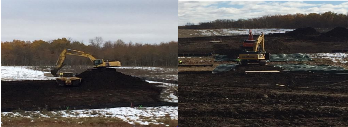
Little Pipestone Creek Prepping for the Bridge Installation
