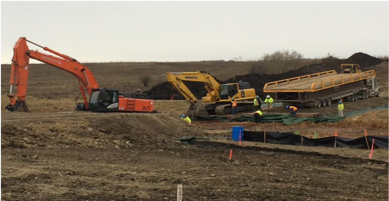
Little Pipestone Creek setting Bridge in place
