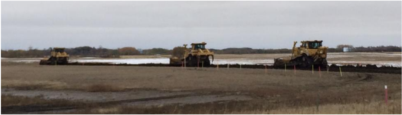
Dozers stripping topsoil
